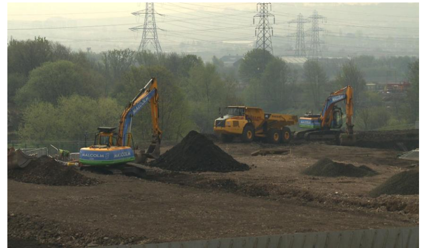
FOUNDATION WORKS UNDERWAY ON GAMES VILLAGE SITE
